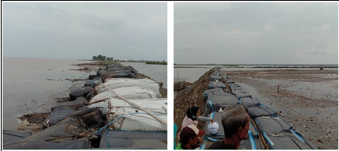
Figure 1. Construction of a pond embankment to withstand coastal erosion aggression.
